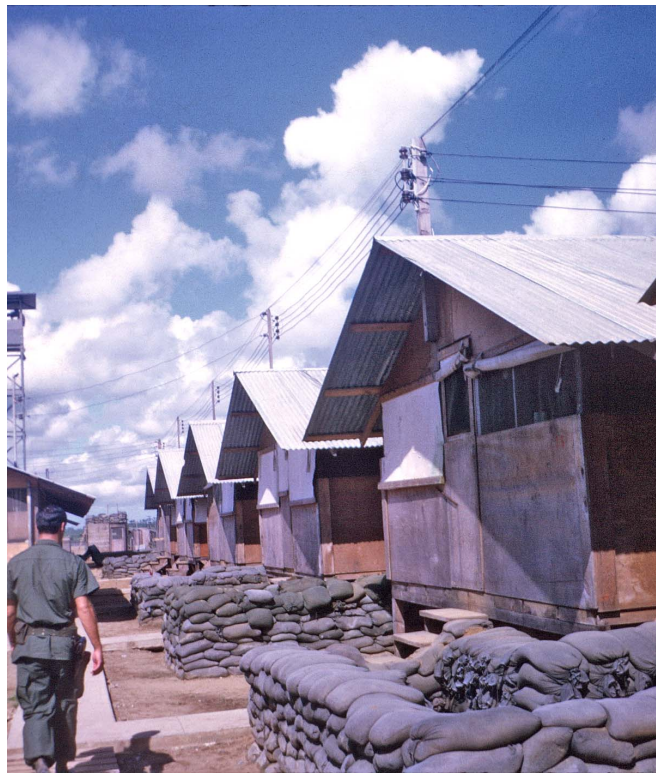
Double rows of sand bags surround the barracks at Solid Anchor
